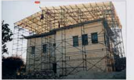
Restorasyon İşleminde Koruma İskelesi Protection During Restoration Works
